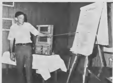
bun, representative of Foxboro Company of Massachusetts. The advanced electronic Process control equipment permits improved display and handling of process control information and can be tied in to any of Lago's present electronic control systems.
